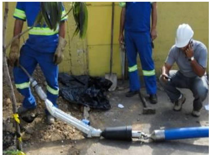
The roller cutter DN 100 mm (4") is assembled with the expander cone and the new HDPE pipe.
