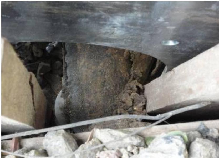
The roller cutter reaches the target pit. The bursting tools are pulled into the front box of the TERRA-EXTRACTOR X 400 and may be disassembled easily.
